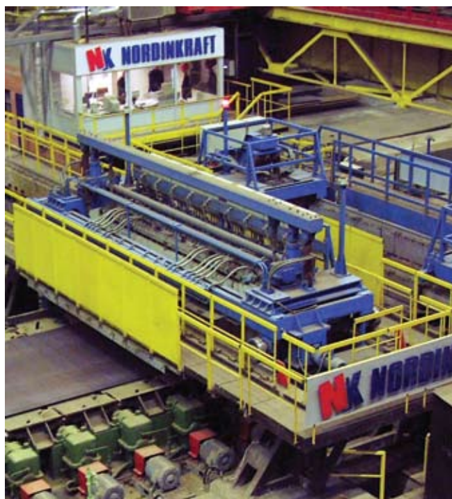
Fig. 10. Plate testing system EMATEST-PL – Plate rolling shop-3, Severstal, Kolpino (Russia).
